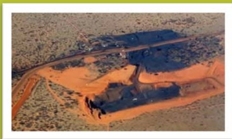
Mine development in progress
